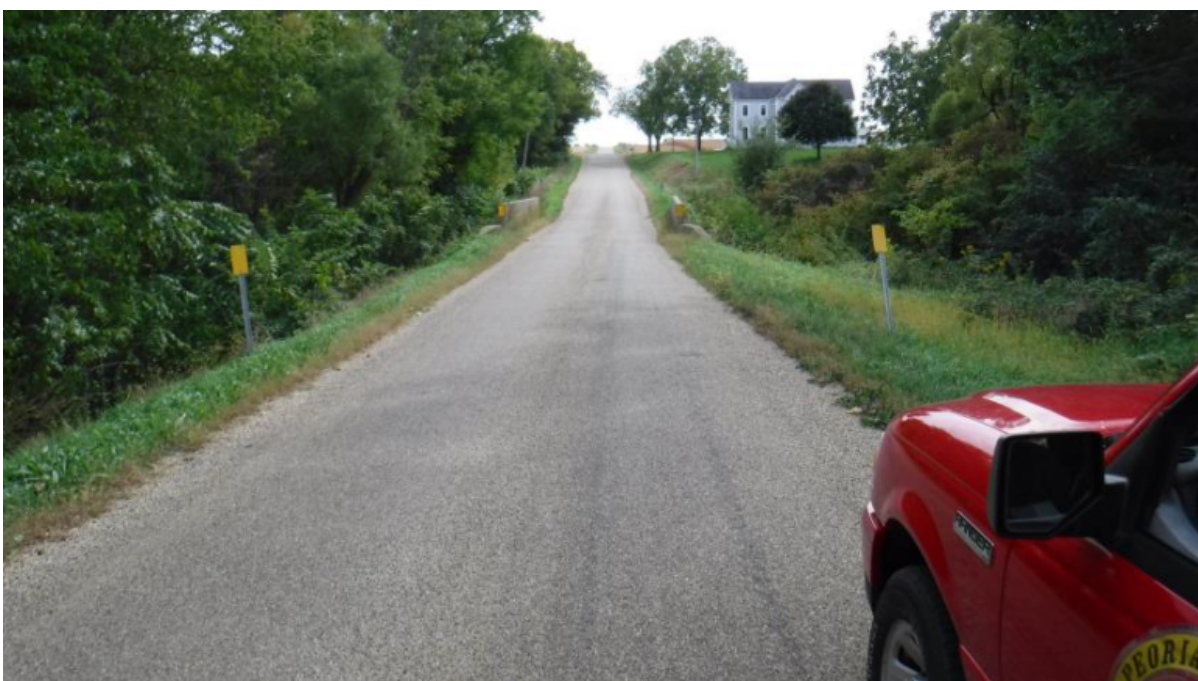
The structure has an ADT rating of 200 cars per day; 12 percent is truck traffic.
