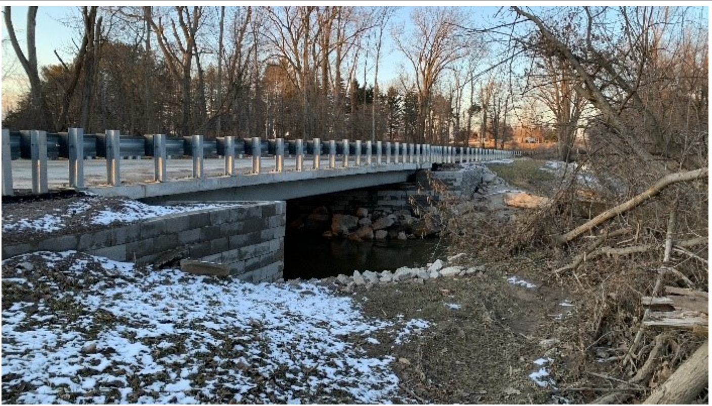
Valmont Structures fabricated the press-brake tub girders for the Orr Road Bridge (Midland County, Michigan) that consists of a precast concrete deck on galvanized steel tub girders.
